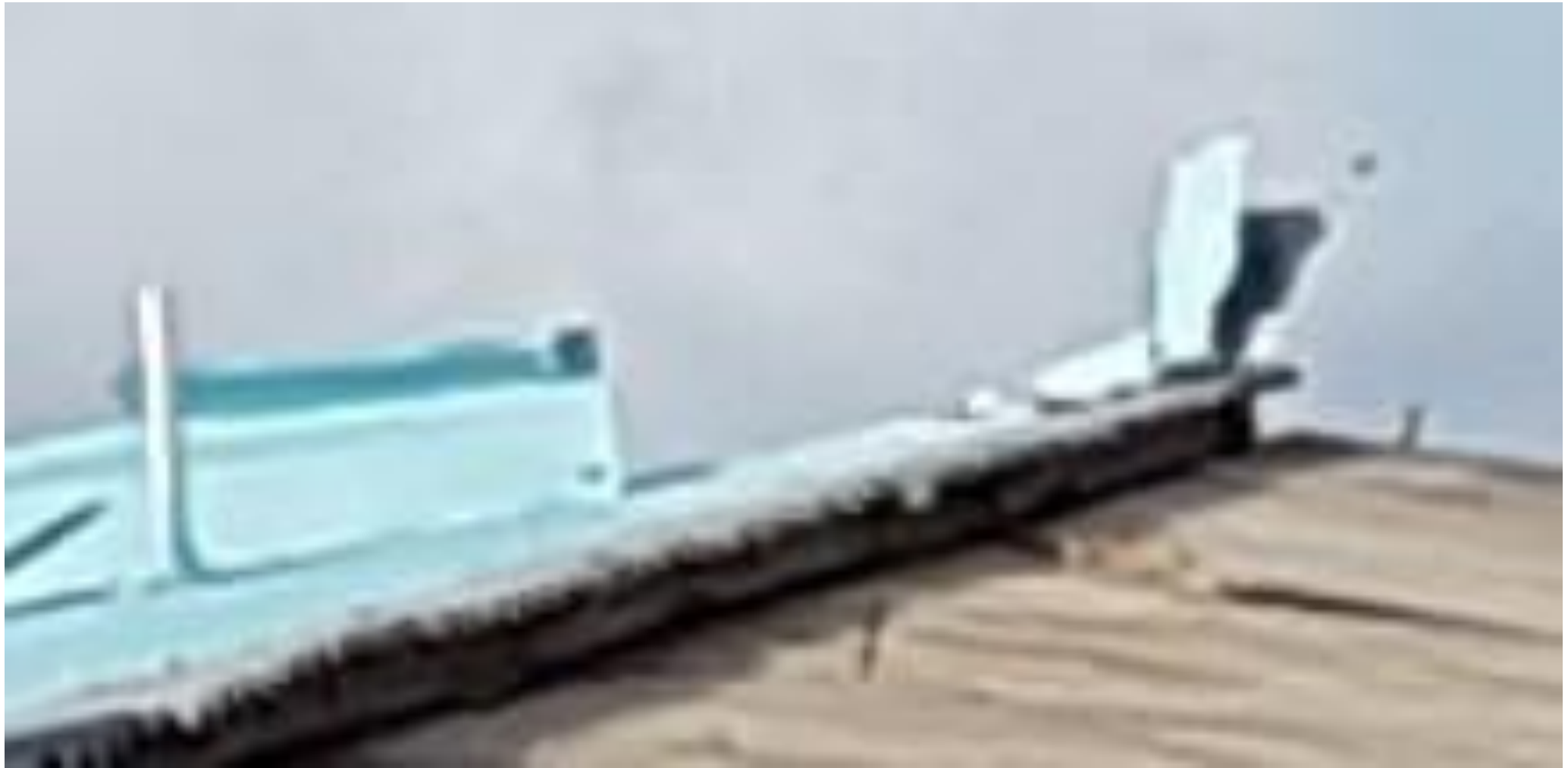
IMAGE 17 –EXAMPLE OF SHEETING TEAROUT
