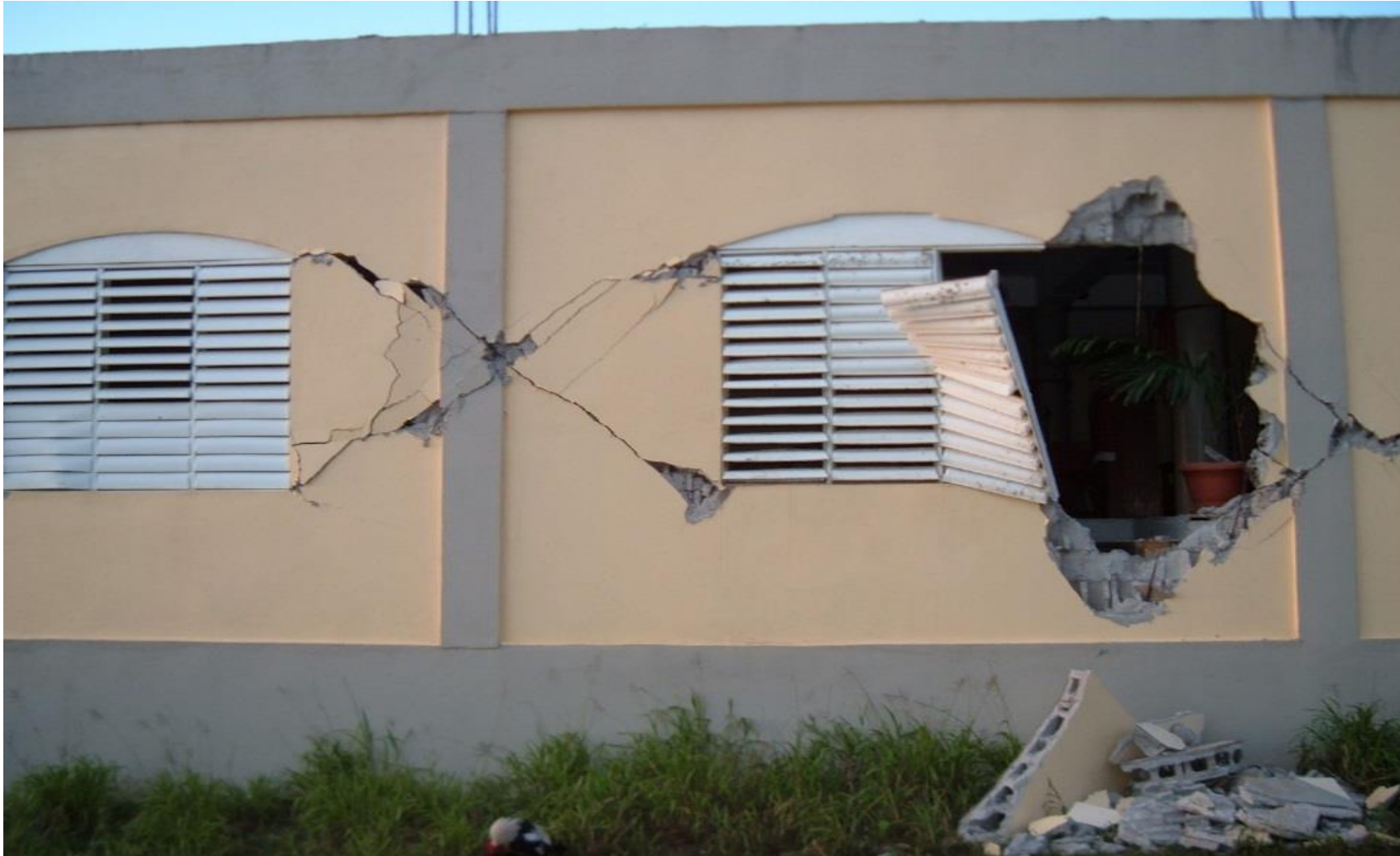
IMAGE 32 – 150 mm RC Masonry Infilled Frame Failure #1 (Dominica Earthquake of 21 November 2004; M_R = 7.0 , 27 km; Fling-type Motion)
