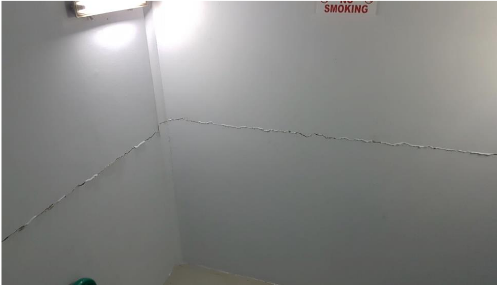
IMAGE 51 - TYPICAL CRACKING OF STAIRWELL CORE WALLS (OTHER SEGMENTS)
