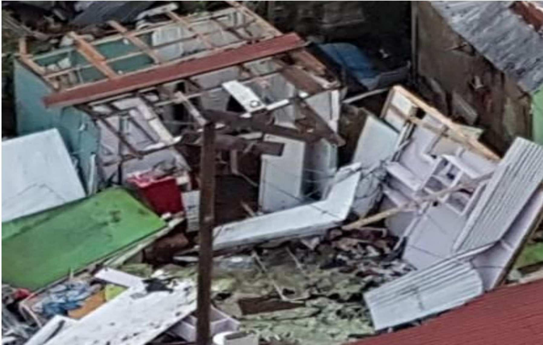
IMAGE 18 –EXAMPLE OF TIMBER OUT-OF-PLANE WALL FAILURE
