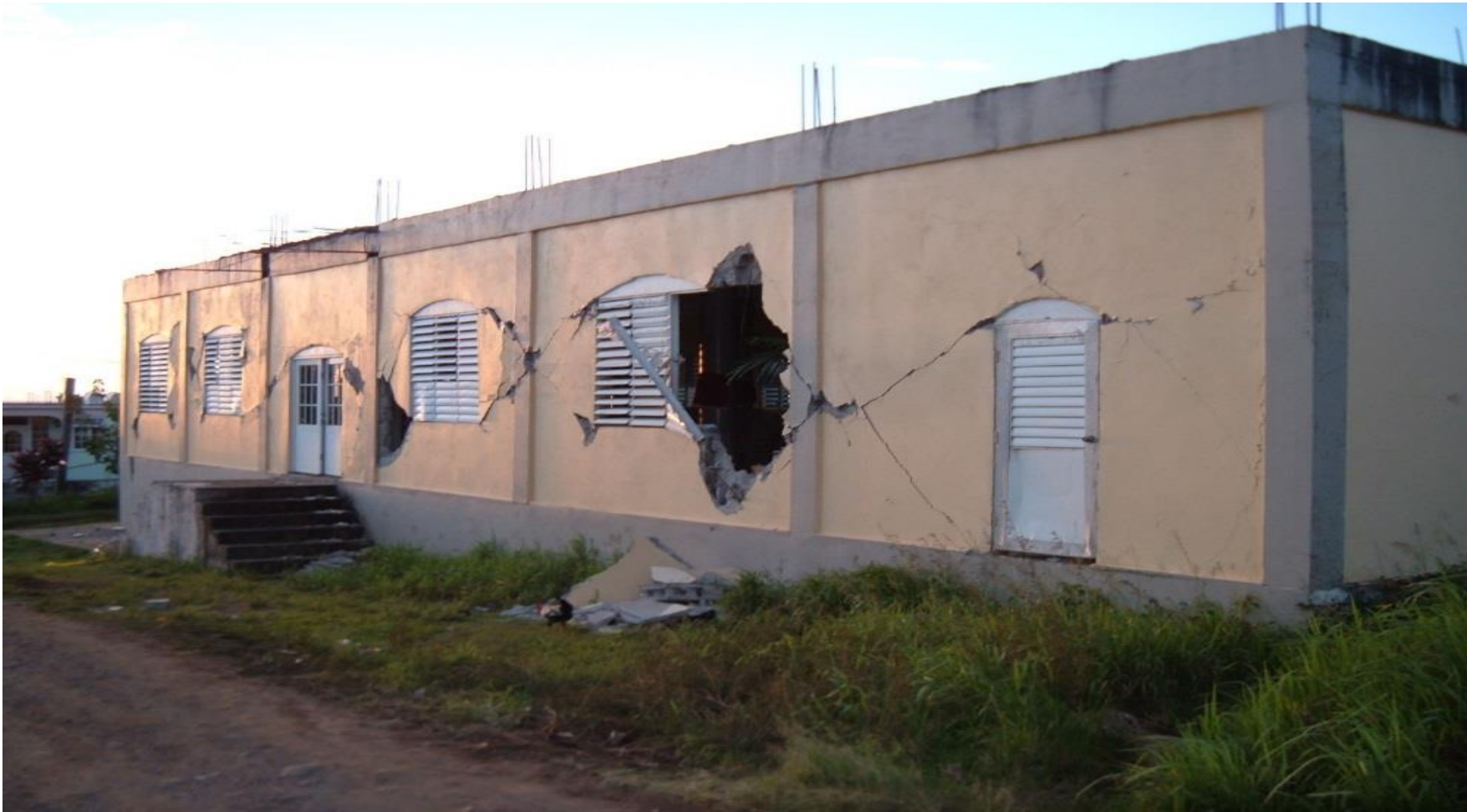
IMAGE 33 – 150 mm RC Masonry Infilled Frame Failure #2 (Dominica Earthquake of 21 November 2004; M_R = 7.0 , 27 km; Fling-type Motion)
