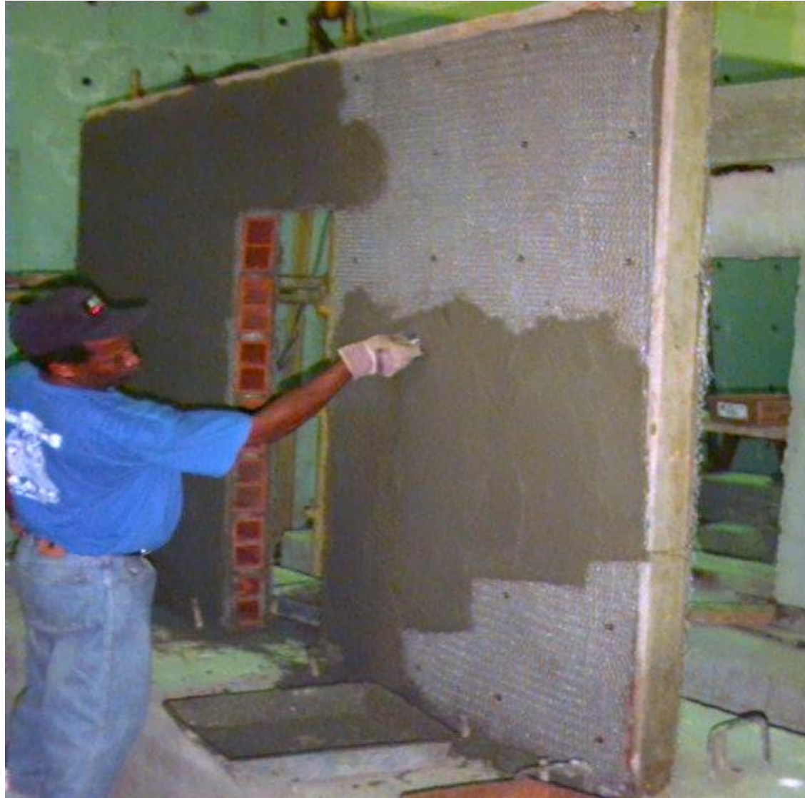
IMAGE 38 – INSTALLATION OF UWI R&D MASONRY WALL RETROFIT TECHNOLOGY
