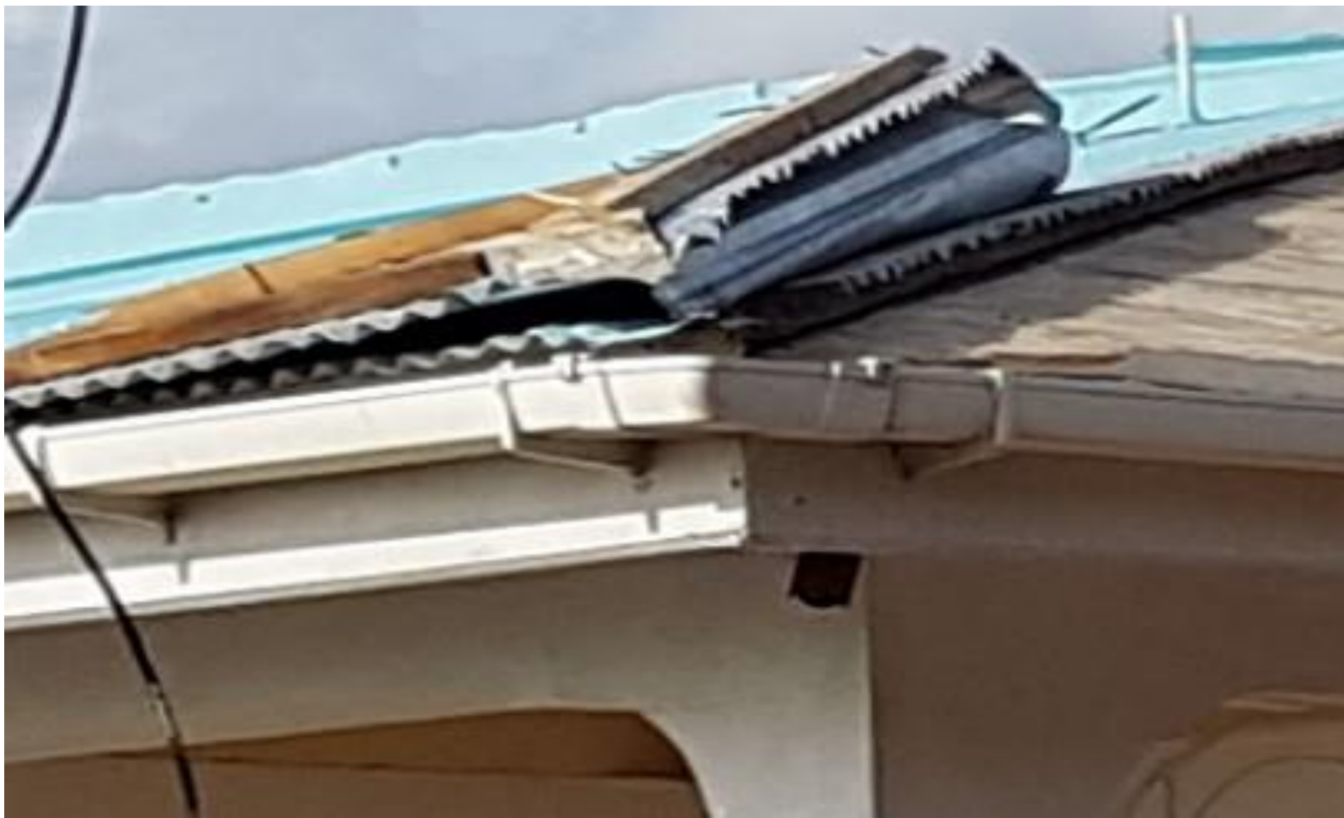
IMAGE 16 –EXAMPLE OF NAIL PULLOUT
