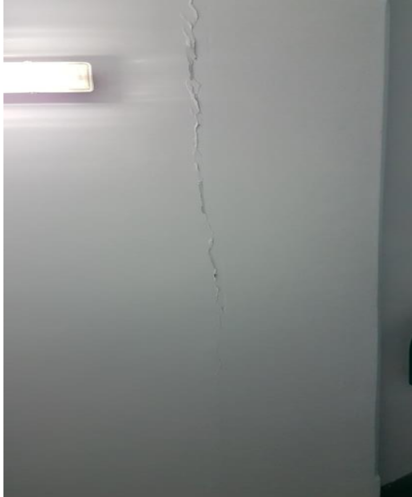
IMAGE 52 - CRACKING AT WALL-COLUMN INTERFACE
